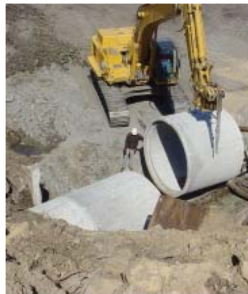
Cover: Concrete pipe under extended lanes and overburden up to 20 feet.
