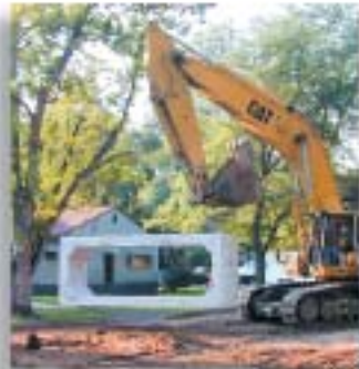
◀ 16-ft. x 5-ft. precast RCB sections replaced a similar-size cast-in-place structure.
