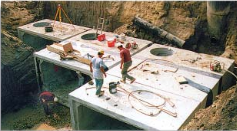
Precast concrete box sections being used for storm water detention.
