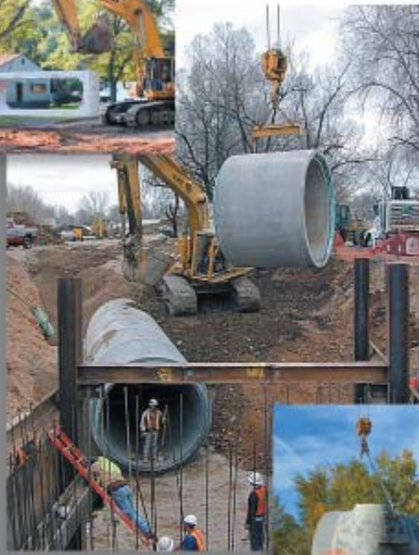
▲ Installation of 108-inch diameter RCP approaches the transition/drop structure.
