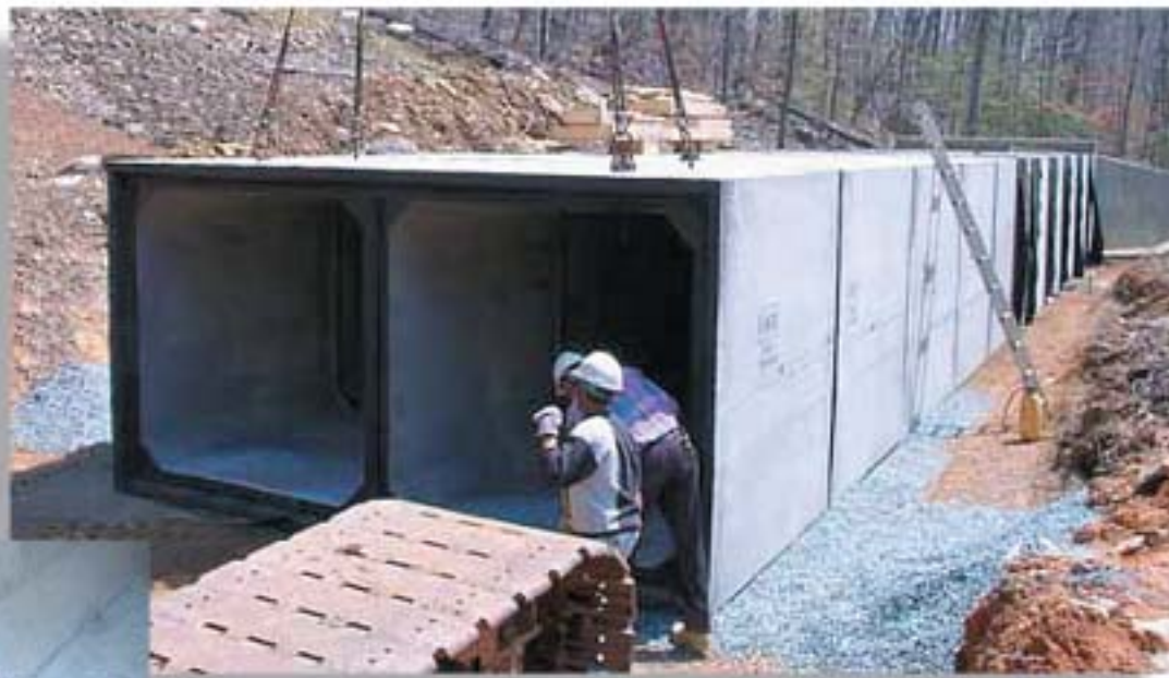
Installation of the 170-foot long twin cell reinforced concrete box culvert was completed in one week.
