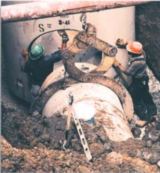
Stringent quality control efforts and exacting installation procedures yielded watertight joints at all manholes.
