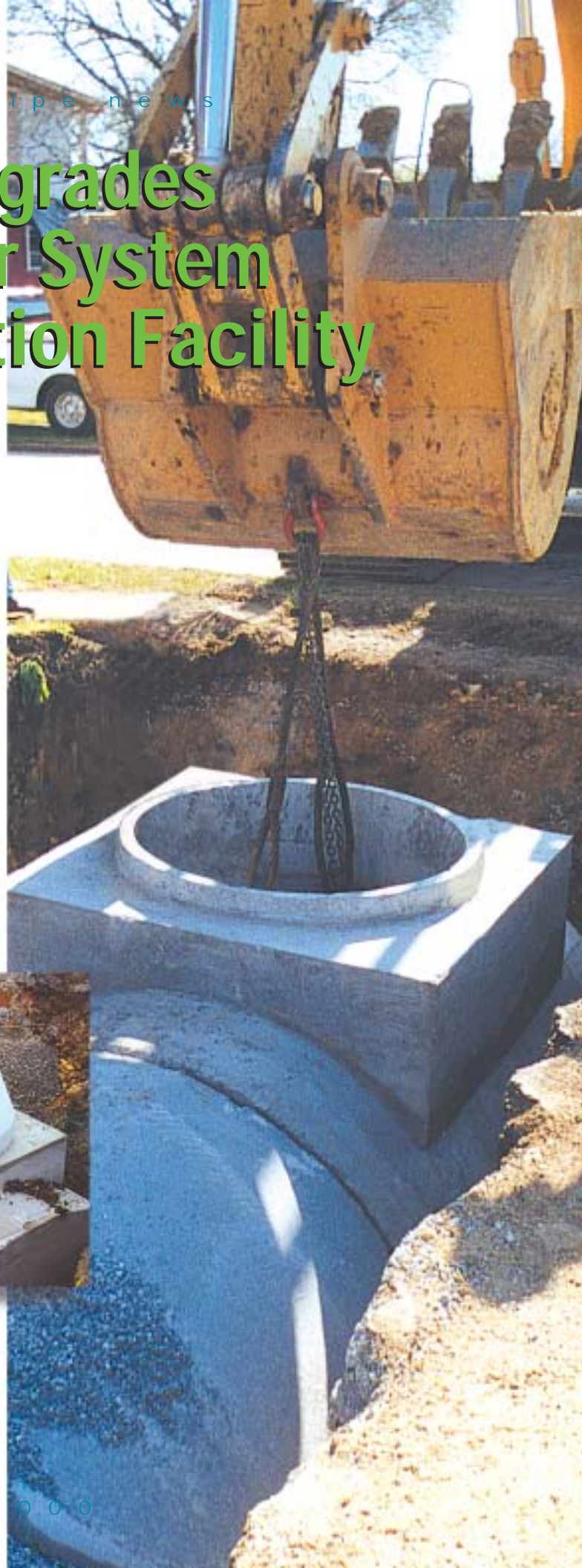
The RCP detention facility will help prevent overtaxing the existing CSO during anticipated redevelopment in the downtown Chattanooga area.
