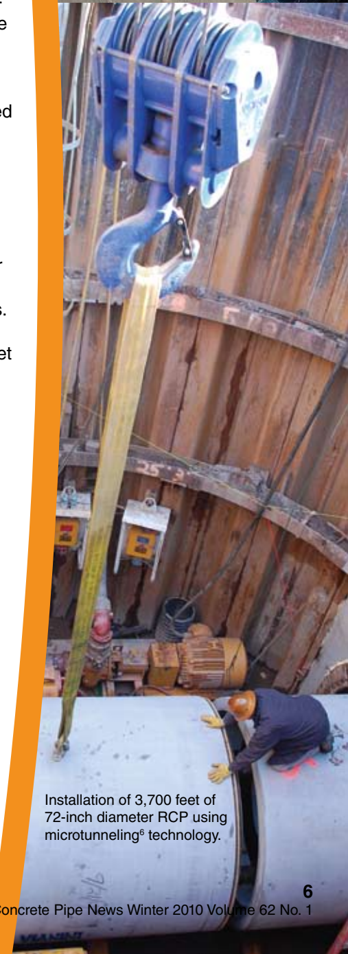
72-inch diameter RCP prepared for installation.
