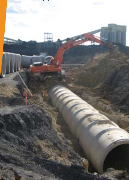
Installation of the mine tunnel in New South Wales, Australia. www.concpipe.asn.au
