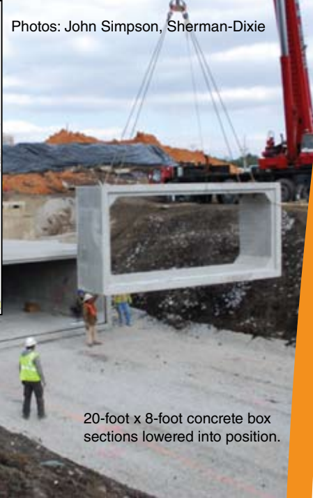
Precast concrete box sections joined with butyl mastic to reduce exfiltration and infiltration.
