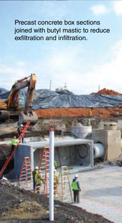
Installed precast concrete box rainwater storage structure ready for backfill with native soil.
