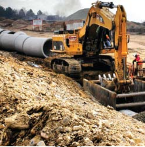
Concrete pipe meets UDOT test requirements after installation.
