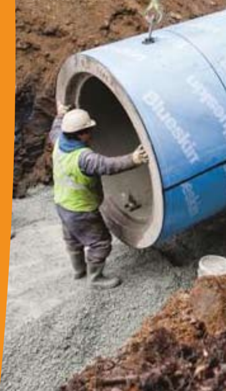
Three-sided box used for pedestrian bridge and support for stream crossing of sanitary sewer.
