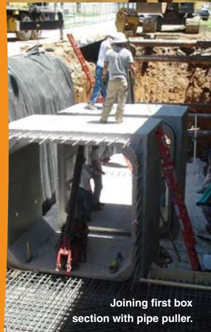
Boxes installed within a narrow alignment.
