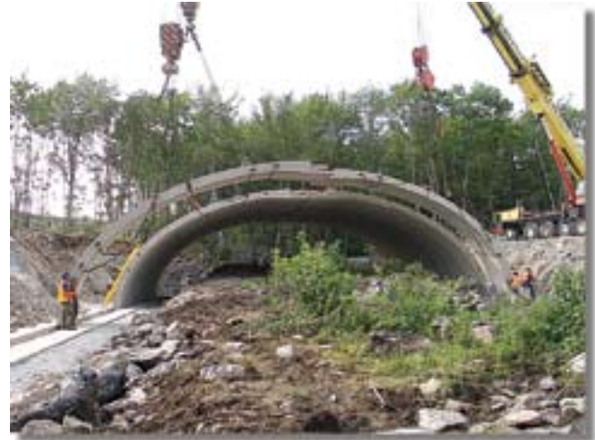
Precast concrete arch product used for stream crossing.
