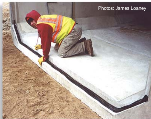
Joint mastic ensures water tightness.
