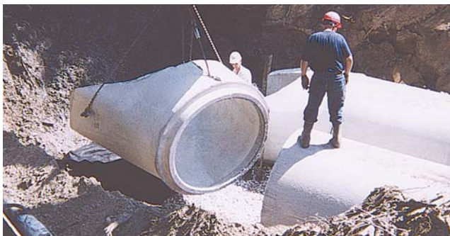
Reinforced precast concrete pipe used as end-of-life solution for failed corrugated metal pipe culvert.
