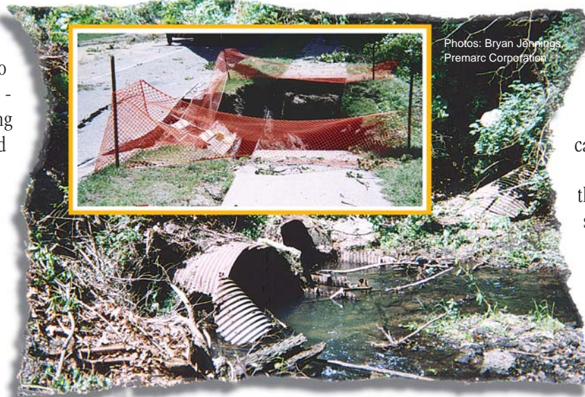
Failed 60-inch CMP culverts replaced with twin 60-inch concrete pipe culvert.
