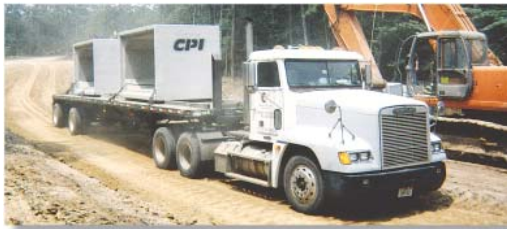
Precast concrete box sections used for double, triple, and quadruple culverts.
