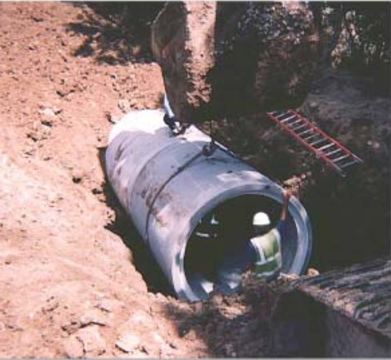
Installation of 72-inch diameter reinforced concrete pipe to carry irrigation water.
