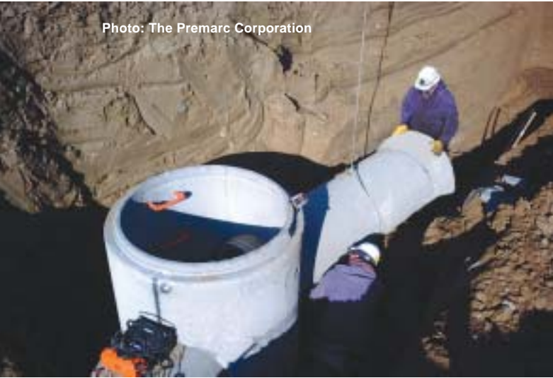
Concrete pipe installed with rubber compound gaskets to resist water and fines infiltration at the joints.
