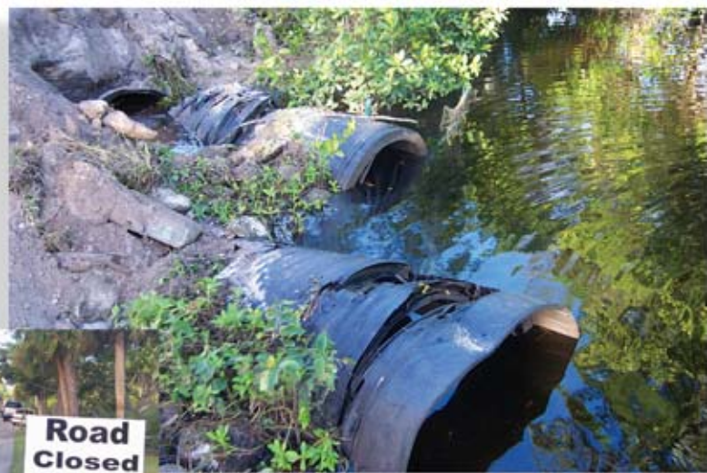
▲ Failed triple run of 48-inch HDPE pipe.
