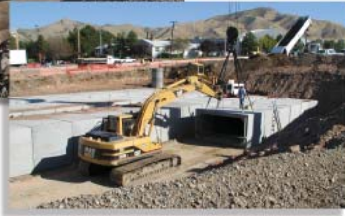
Stormwater controlled with four rows of box sections.
