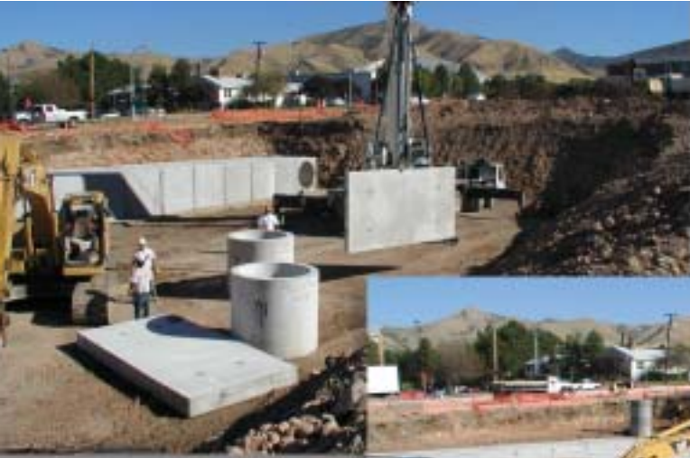
Stormwater controlled with four rows of box sections.
