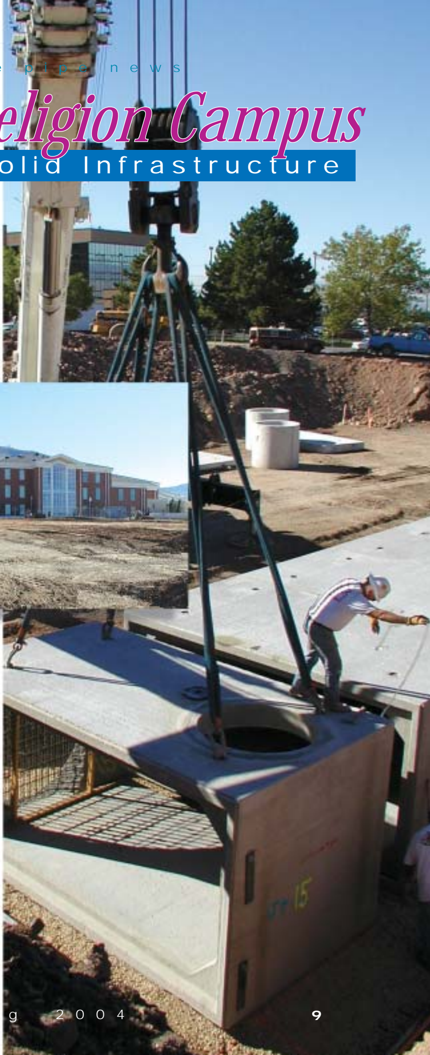
RCP specification changed to precast concrete boxes.
