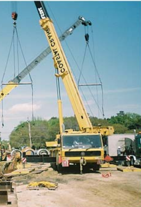
Installation of twin 60-inch diameter RCP storm sewer.
