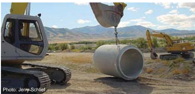
54-inch pipe being transported to the trench.
