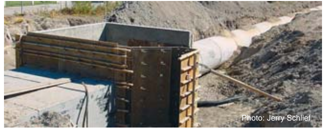
Casting of a transition between the 54-inch pipe and the 11-foot x 4-foot box section.
