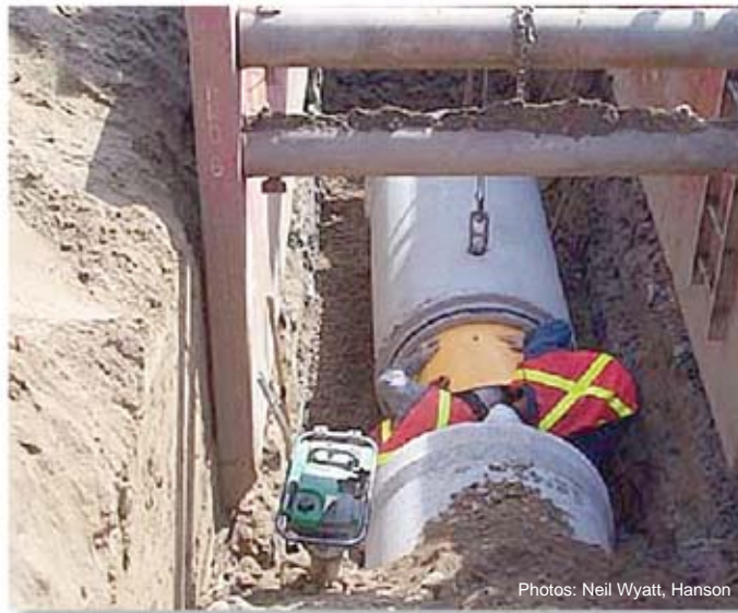
Installation of 36-inch reinforced concrete pipe.
