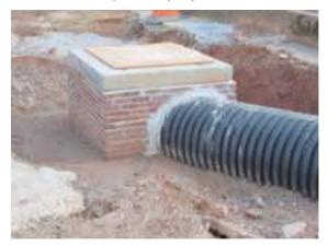
7.11 Field Monitoring—Compliance with contract documents with respect to pipe installation, including trench depth, grade, water conditions, foundation, embedment and backfill materials, joints, density of materials in place, and safety, should be monitored by the engineer at a frequency appropriate to project requirements.
