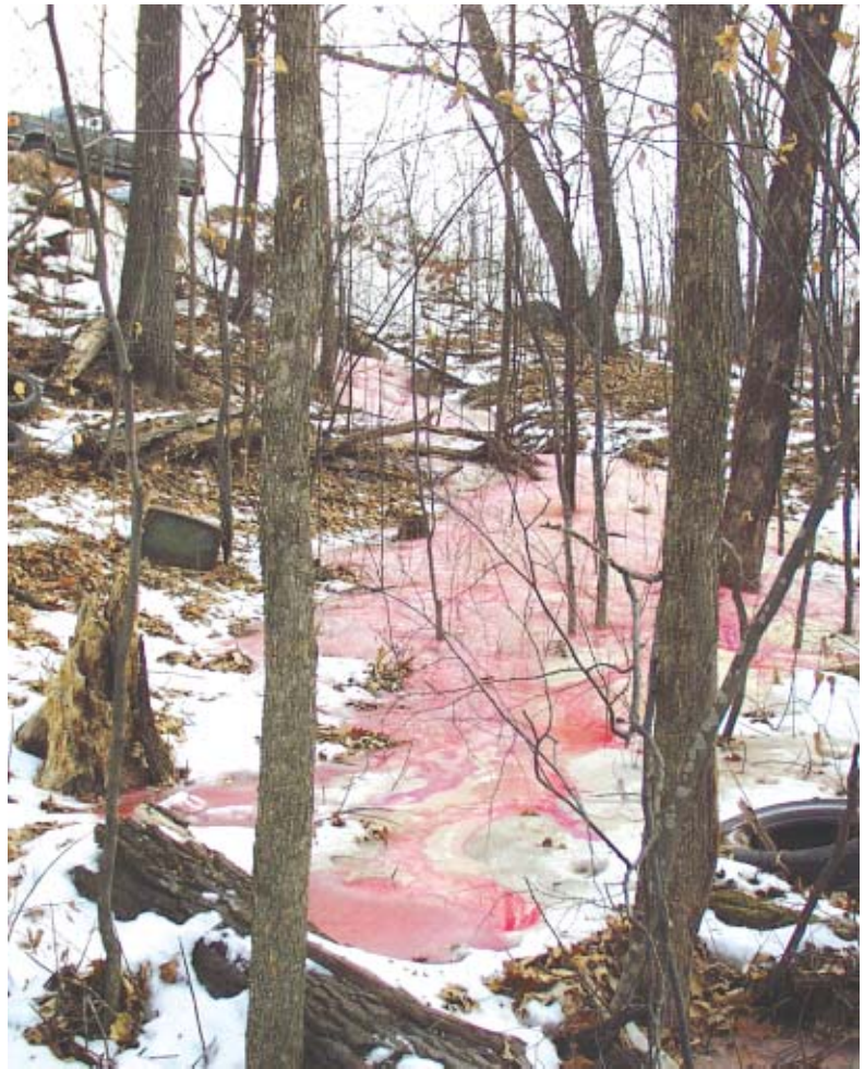
One of the many areas where trace dyes leaked from the HDPE pipeline during testing of the pipeline during the winter months.
