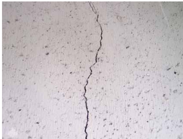
Exhibit 109. Minor longitudinal crack with efflorescence.
