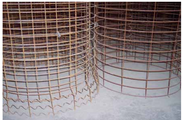
Circumferential steel provides the structural component of the completed steel cage
