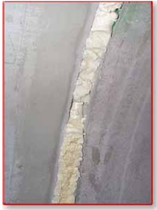
Internal Chemical Grouted Joint
