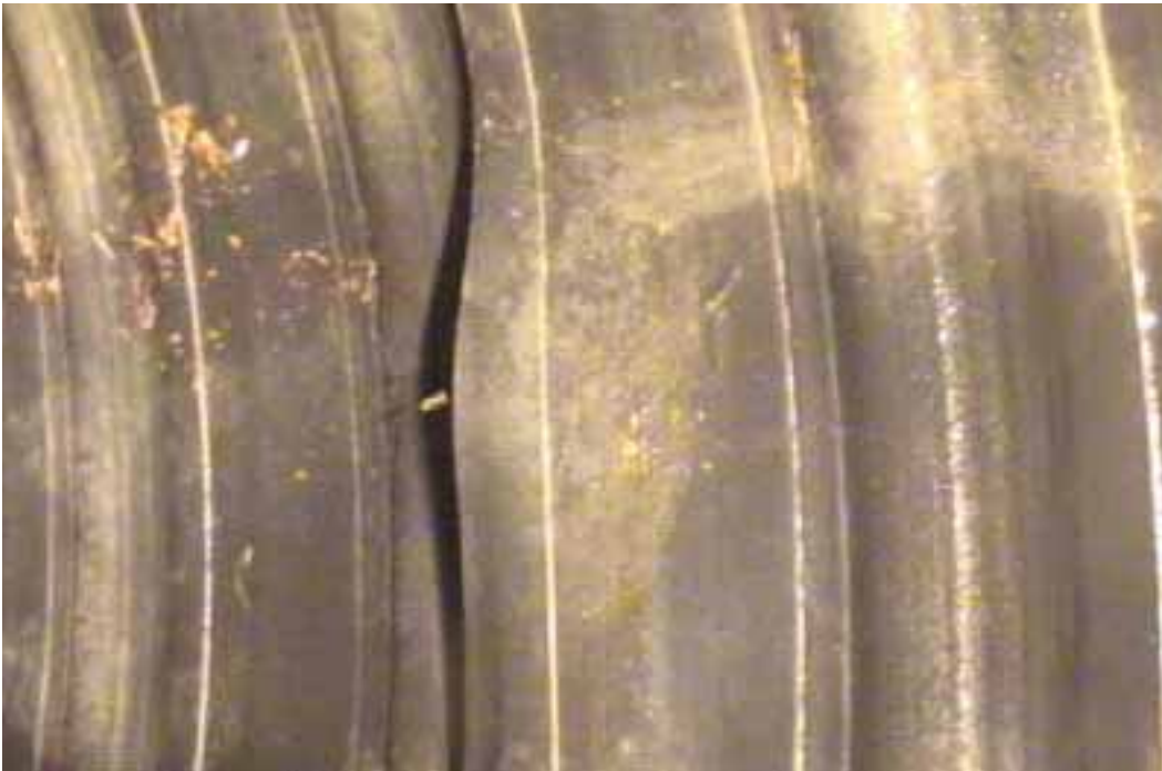
Figure 423 Cracking/fracture failure for Pipeline No. 8 (Site No. 7: West Island Road)
