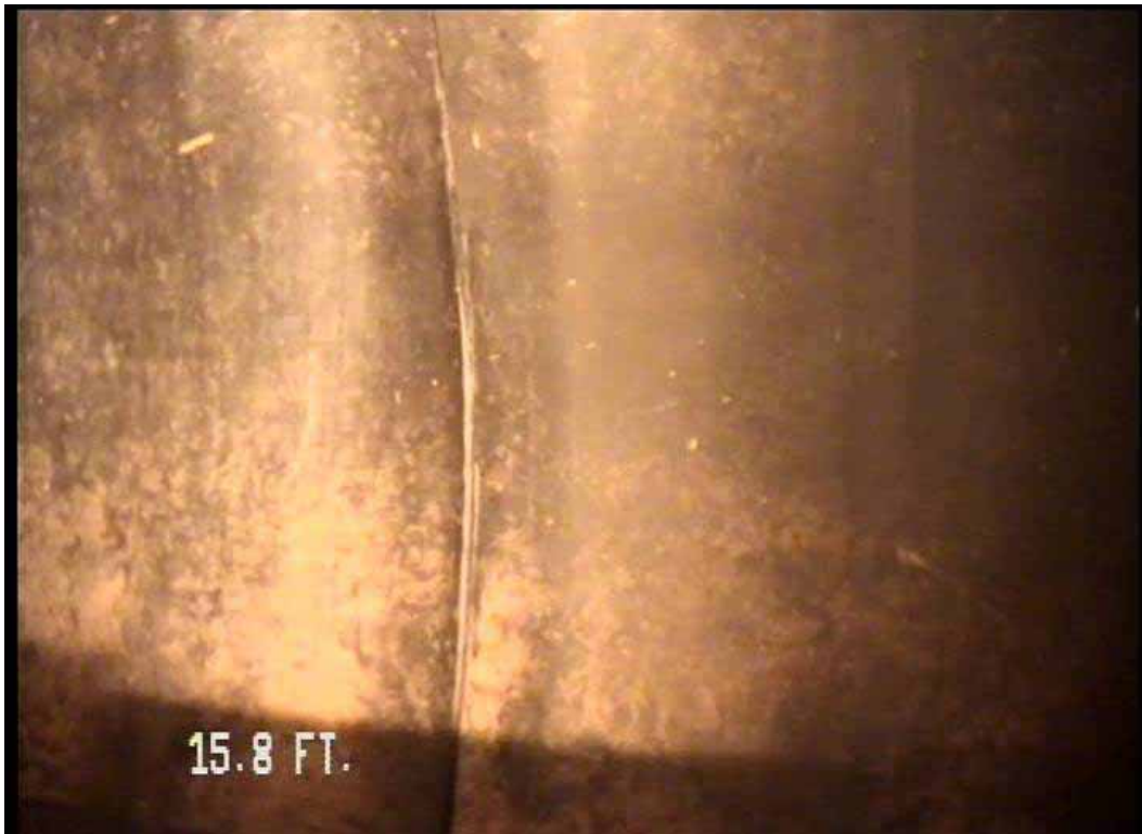
Figure 511 View of the joint for pipeline No. 6 (Site No. 1: Orlando)
