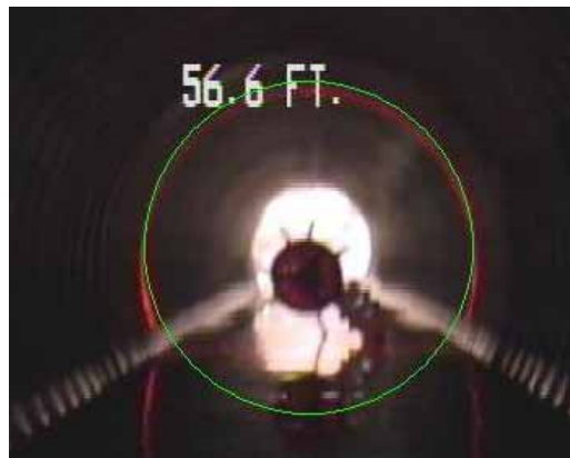
Figure 35 Horizontal and vertical deformation of the pipeline No. 9 (Site No. 5: Houston – Riley Fussel)
