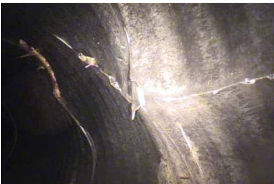
Figure 52 Major joint, inverse curvature and cracking/fracture failures for pipeline No. 20 (Segment 1) (Site No. 8: Houston – Fennell)
