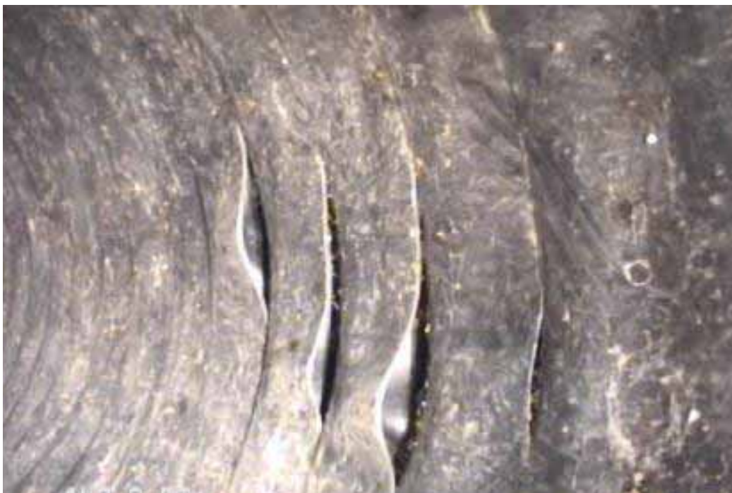
Figure 291 Cracking/fracture failure for Pipeline No. 7 (Site No. 1: Route 101)
