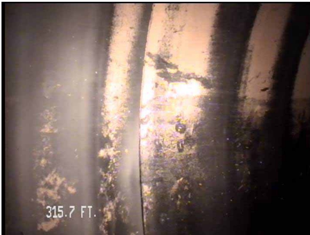
Figure 501 View of the joint for pipeline No. 3 (Site No. 1: Orlando)
