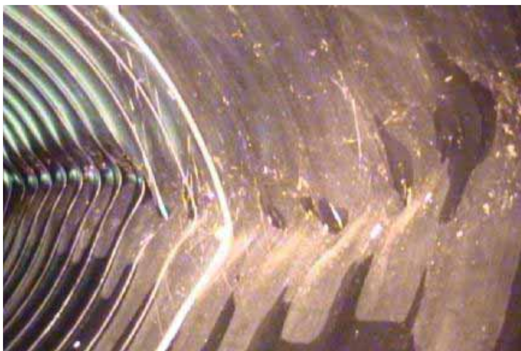
Figure 450 Buckling and corrugation growth failure for Pipeline No. 21 (Site No. 11: Houghton County-North Laird Heights)
