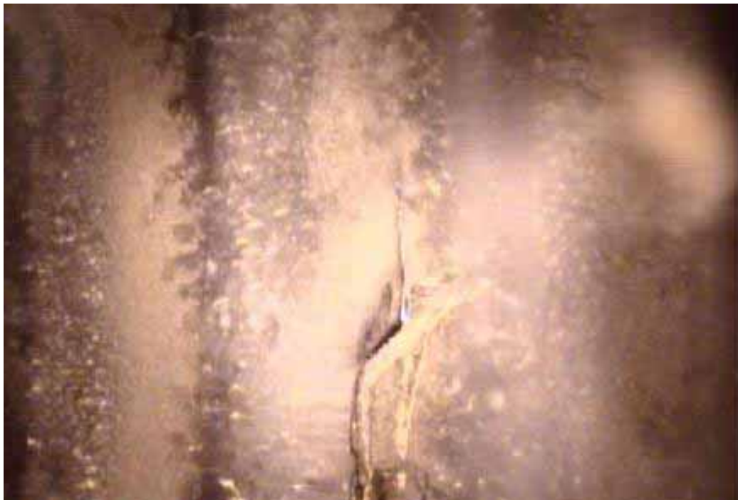
Figure 463 Cracking/fracture failure for Pipeline No. 24b (Site No. 13: Burlinghame Avenue)
