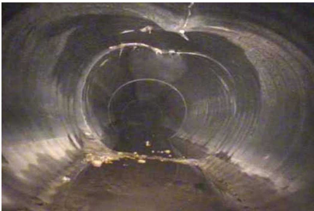
Figure 52 Major joint, inverse curvature and cracking/fracture failures for pipeline No. 20 (Segment 1) (Site No. 8: Houston – Fennell)
