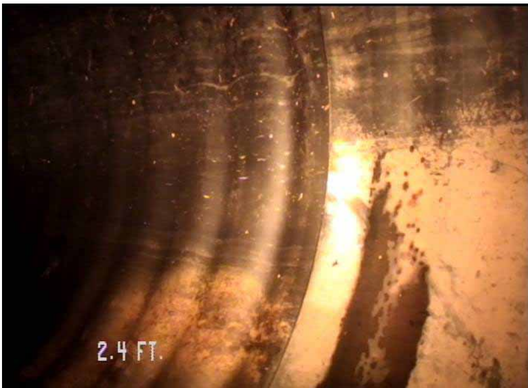
Figure 534 View of the joint for pipeline No. 9 (Site No. 1: Orlando)
