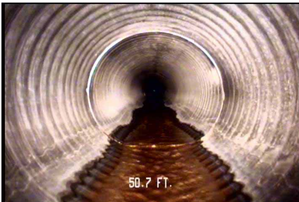
Figure 547 View of the corrugation growth failure and dips in line and grade for pipeline No. 10 (Site No. 2: Apopka)
