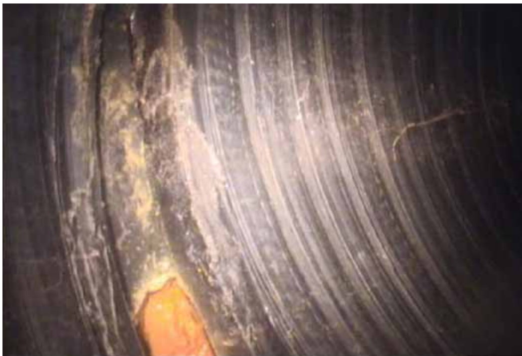
Figure 98 View of major joint displacement failure for pipeline No. 11 (Site No. 6: Rockingham – Love Ln)
