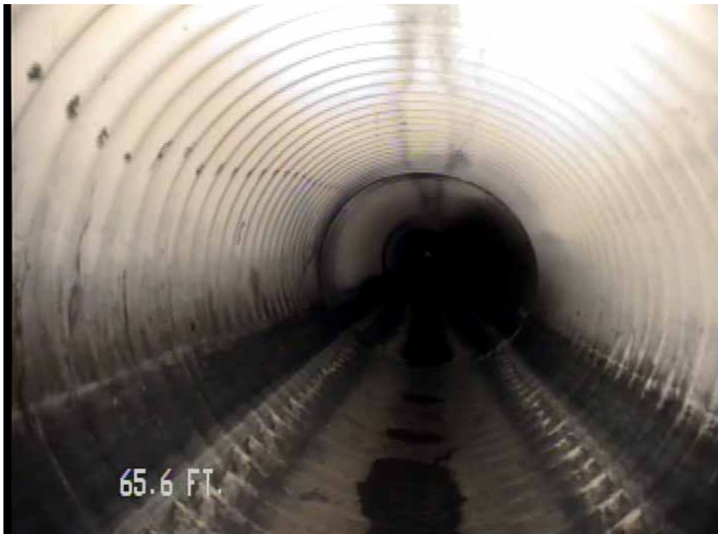
Figure 555 View of corrugation growth failure for pipeline No. 11 (Site No. 2: Apopka)
