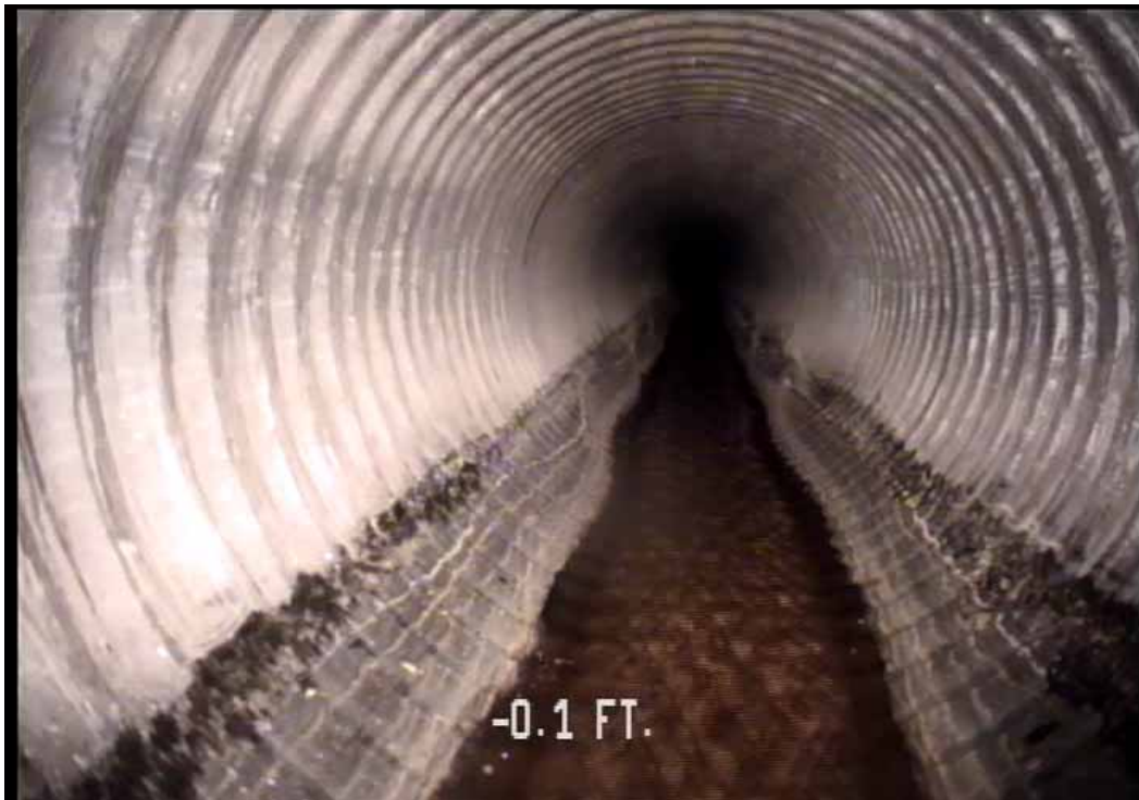
Figure 542 View of the corrugation growth failure for pipeline No. 10 (Site No. 2: Apopka)
