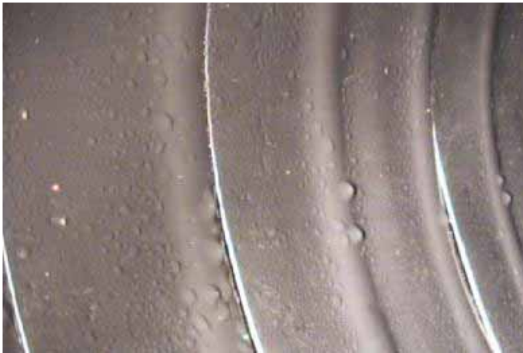
Figure 346 Cracking/fracture failure for Pipeline No. 23 (Site No. 2: Route 36)
