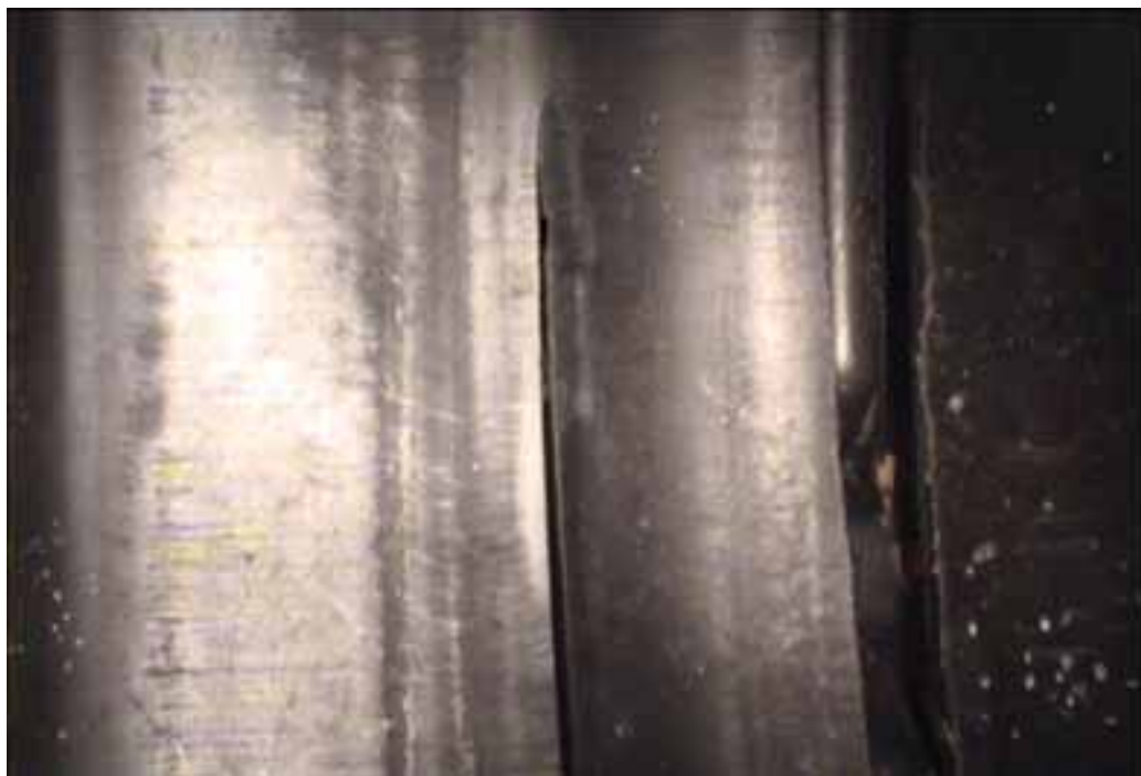
Figure 244 Cracking failure for pipeline No. 11 (Site No. 3: Franklin County – Route FF)
