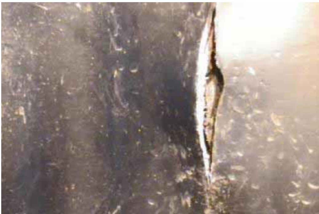
Figure 305 Cracking/fracture and inverse curvature failure for Pipeline No. 9 (Site No. 1: Route 101)
