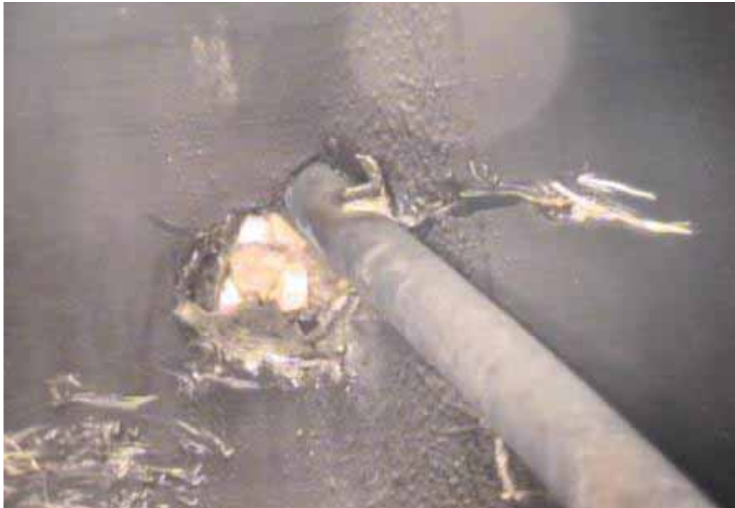
Figure 219 View of pipe intrusion for pipeline No. 6 (Site No. 1: Lenexa)
