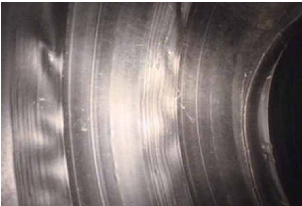
Figure 23 Buckling failure for pipeline No. 1 (Site No. 1: San Antonio - HW 1604 and 1560)
