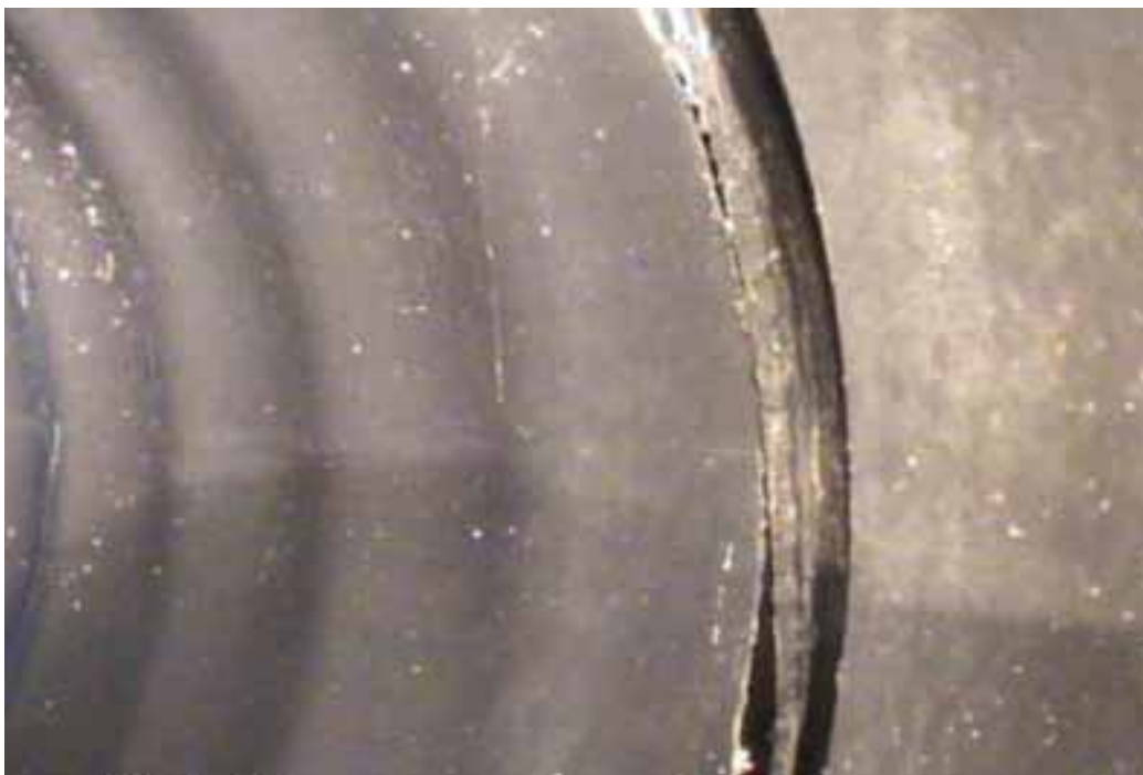
Figure 347 Cracking/fracture and corrugation growth failure for Pipeline No. 23 (Site No. 2: Route 36)
