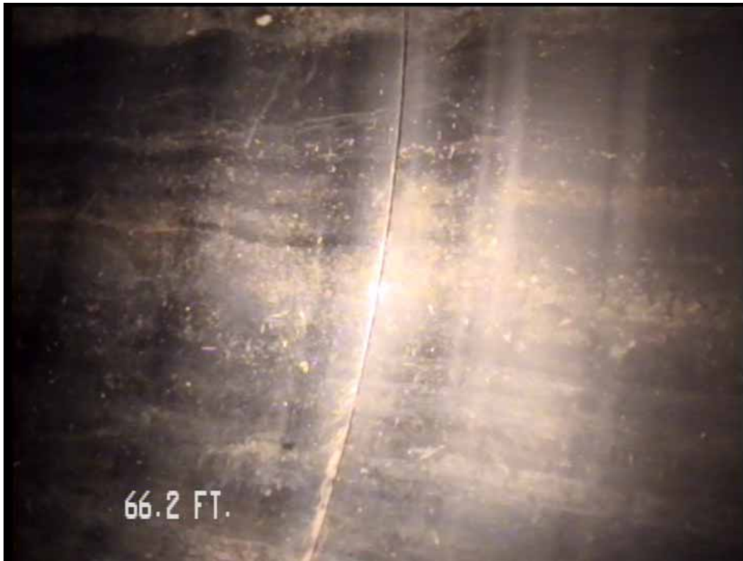
Figure 528 View of joint for pipeline No. 8 (Site No. 1: Orlando)
