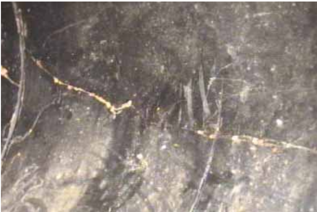
Figure 308 Cracking/fracture failure for Pipeline No. 10 (Site No. 1: Route 101)
