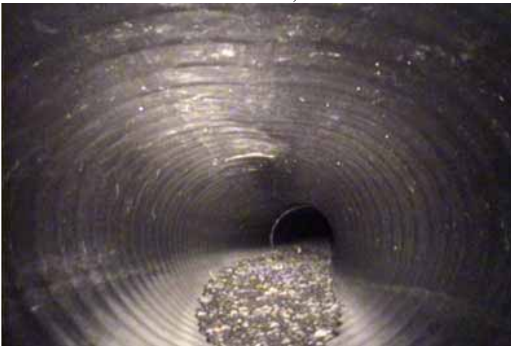
Figure 146 View of major joint displacement failure for pipeline No. 16 (Site No. 6: Winchester)
