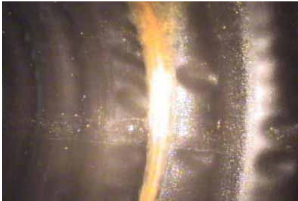
Figure 432 Buckling and corrugation growth failure for Pipeline No. 13 (Site No. 8: Kinross Road)
