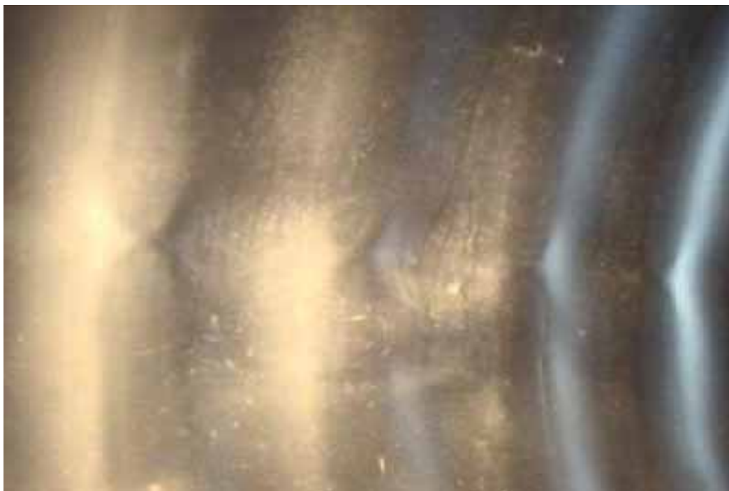
Figure 386 Buckling and corrugation growth failure for Pipeline No. 10 (Site No. 2: Silver Creek Parkway)
