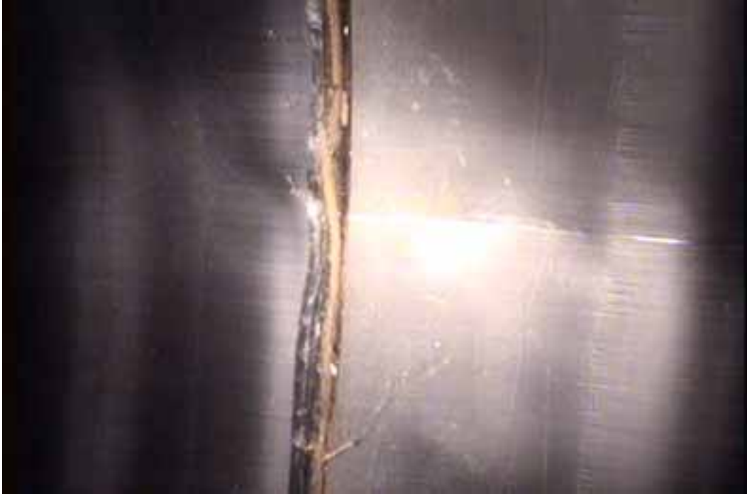
Figure 150 View of buckling failure for pipeline No. 16 (Site No. 6: Winchester)
