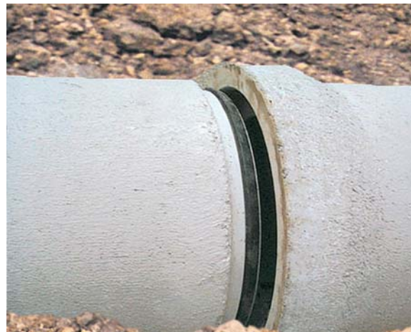
Performance Based — Rubber gasketed concrete pipe joints meet the stringent requirements of ASTM C 443
