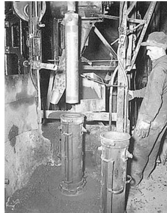
Early production of small diameter concrete drainage tile using a mechanized process. Photo: Courtesy of American Concrete Pipe Association
